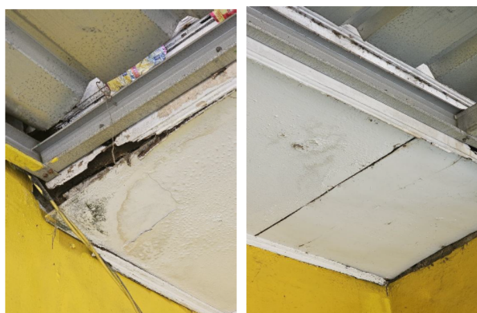
Figure 5. Roof-to-wall joint problems
