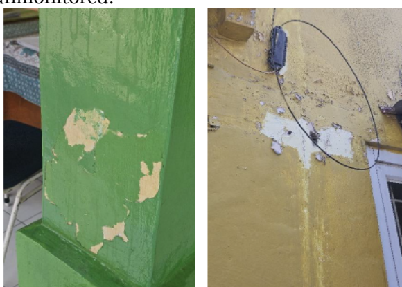
Figure 3. Peeling paints indoor and outdoor
