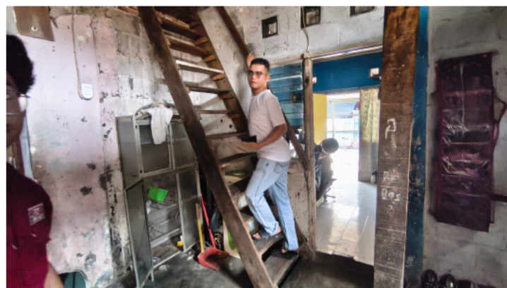
Figure 8. Black molds on walls (Source: Authors' documentation)
