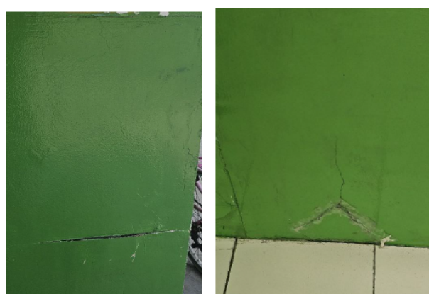
Figure 4. Structural cracks
