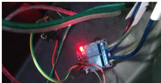
Gambar 6. Kondisi Relay 1 On, Relay 2 Off
