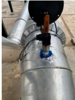
Gambar 6. Pressure Sensor Sistem PCW
