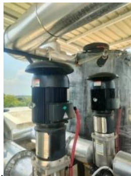
Gambar 2. Pump Sistem PCW
