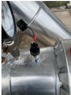
Gambar 7. Temperature Sensor Sistem PCW
