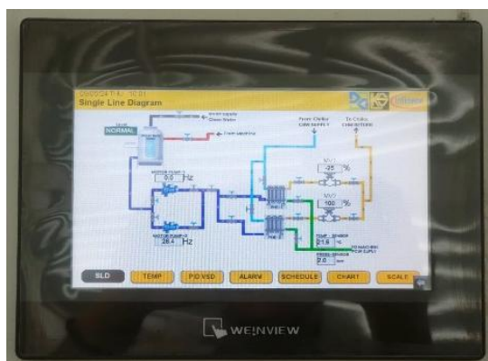
Gambar 9. Single Line Diagram (SLD) Sistem PCW
