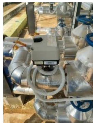
Gambar 5. Motorize Valve Sistem PCW
